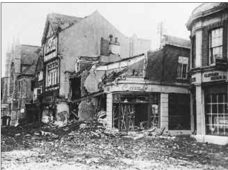
58 Chapel Road, Worthing, September 1940.
