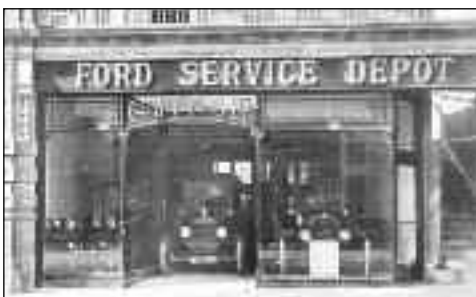
The Ford Depot at Terminus Buildings, Eastbourne.
