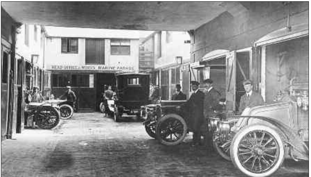
Grange Road lock-up garages opened in 1908.
