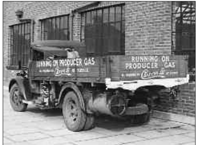
With a shortage, and restrictions on the use of fuel, this 1942 Morris Commercial had been converted by Caffyns to run on 'Producer Gas'.
