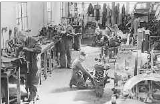
Military vehicles undergoing repair at Hove.
